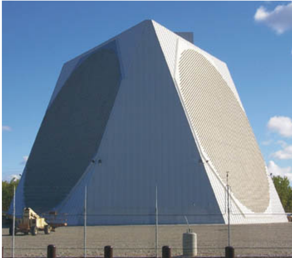
US Air Force 27 m Diameter PAVE PAWS Radar (Alaska) for Missile Defense
